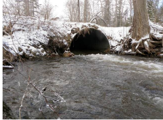
Upgraded culverts can mitigate flooding problems by increasing the flow capacity of streams as they pass under roadways.
