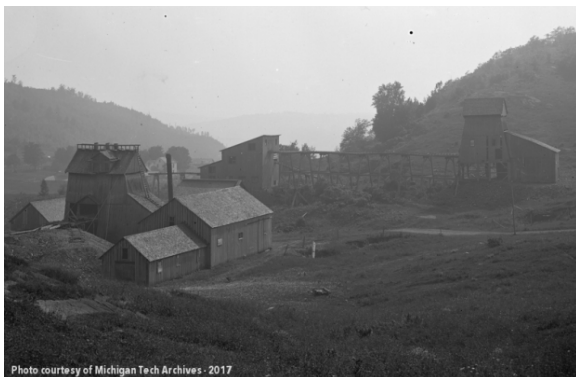
Wooden shaft-houses and several other buildings at National Mine in Rockland (Source: MTU Archives )
