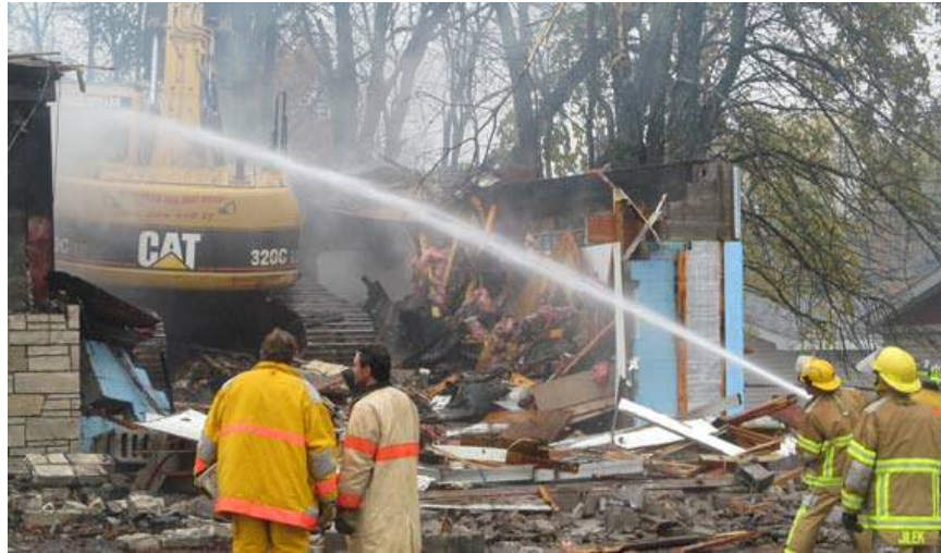
Firefighters spray water on the back portion of the Bergland Foods Store after being destroyed in a fire on October 18, 2013 (Photo: Cortney Ofstad/Daily Globe) 32
