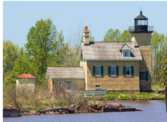
Ontonagon Lighthouse (Source: rossograph , is licenced under CC By-SA 4.0)
