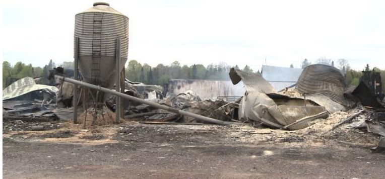
Pelkie Barn destroyed after structural fire on May 27, 2019 (Source: Upper Michigan Source)
