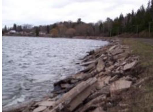
Riprap protects the shoreline from erosion along the Village of L'Anse Waterfront.
