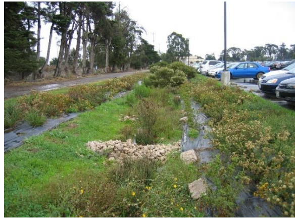
Bioswales are vegetated, or mulched channels that provide treatment and retention as they move stormwater from one place to another. Vegetated swales slow, infiltrate, and filter stormwater flows. As linear features, they are particularly well suited to being placed along streets and parking lots.
