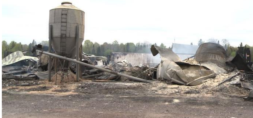
Pelkie Barn destroyed following structure fire, May 27, 2019 (Source: Upper Michigan Source)
