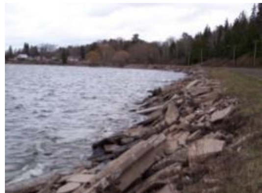
Riprap protects the shoreline from erosion along the Village of L’Anse Waterfront.
