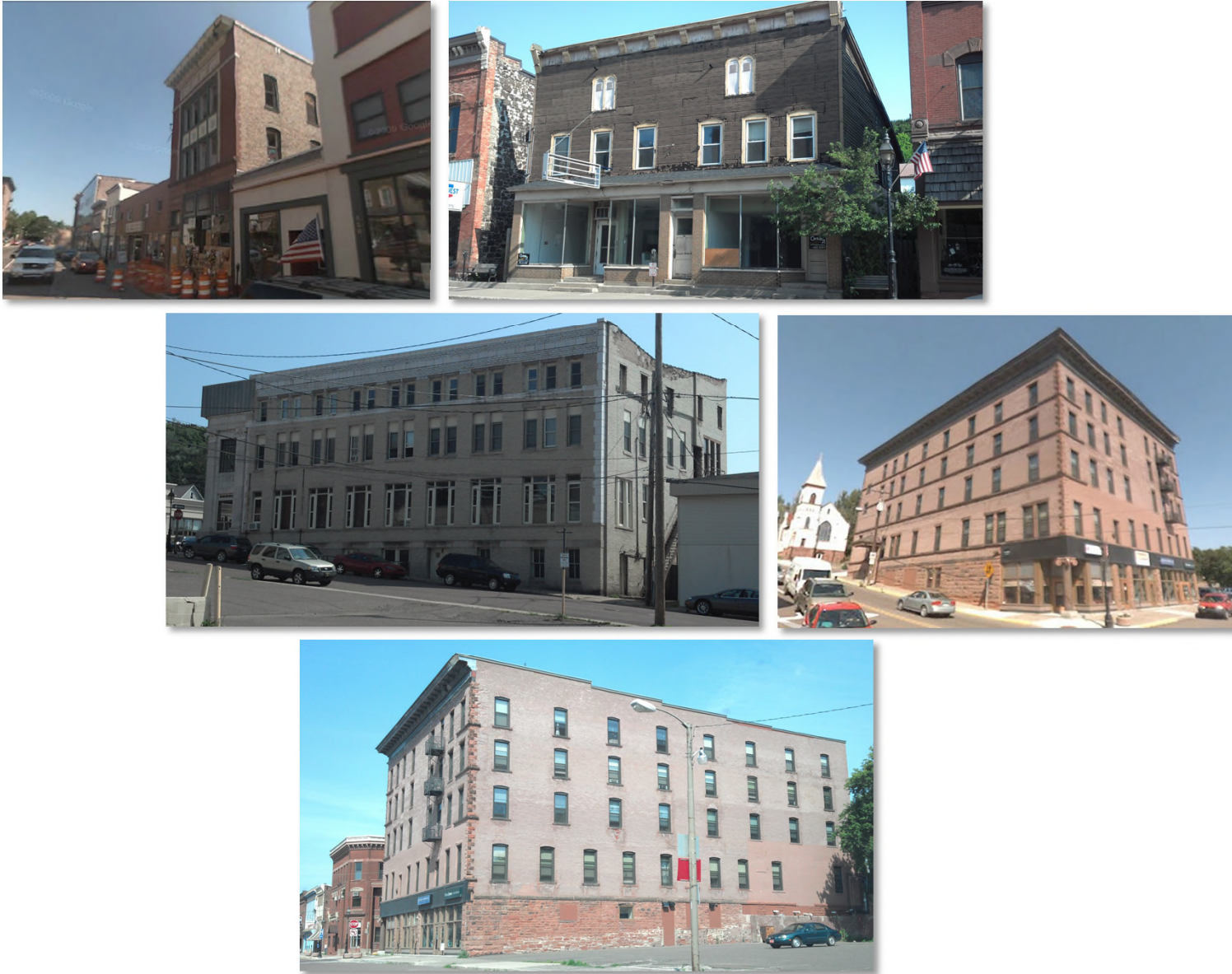
Photo credit (above): Original photos by LandUse|USA; 2016 © with all rights reserved.
