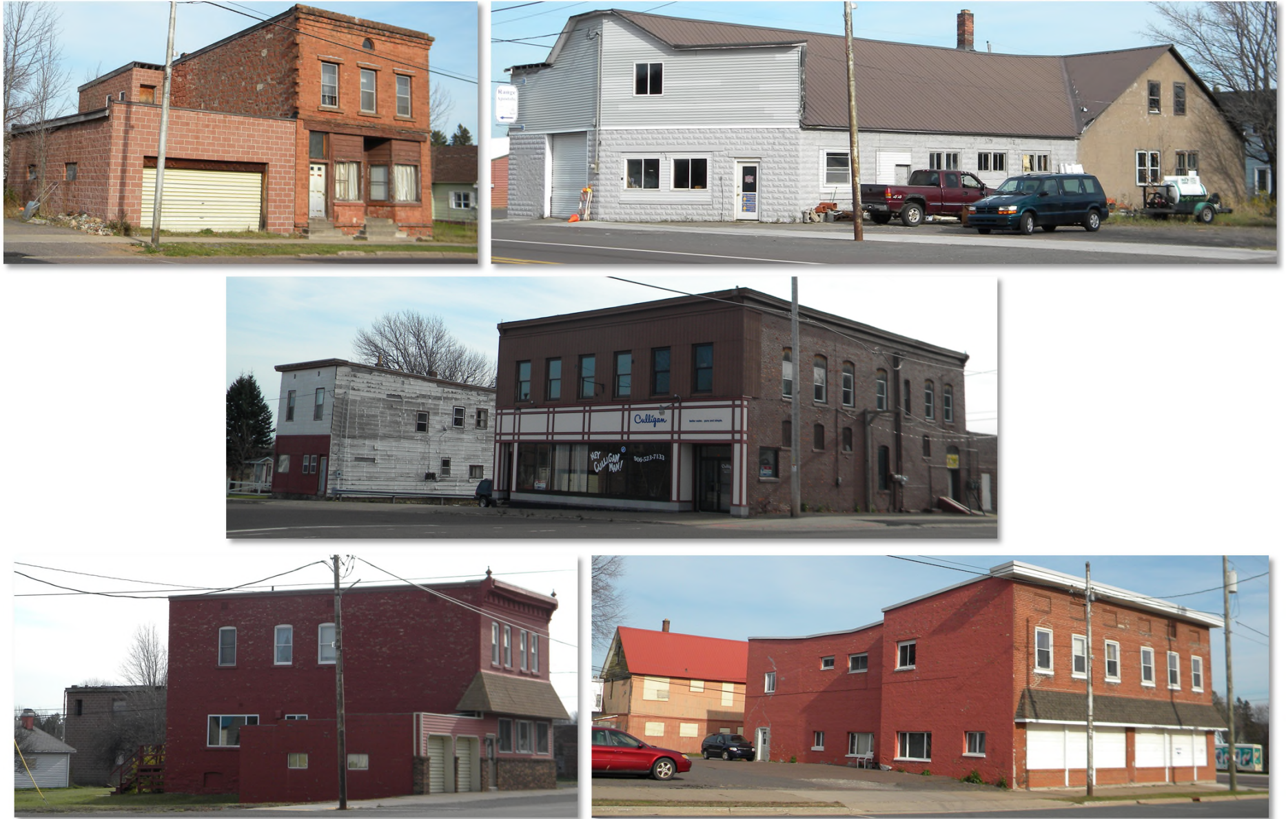
Photo credit (above): Original photos by LandUse|USA; 2016 © with all rights reserved.
