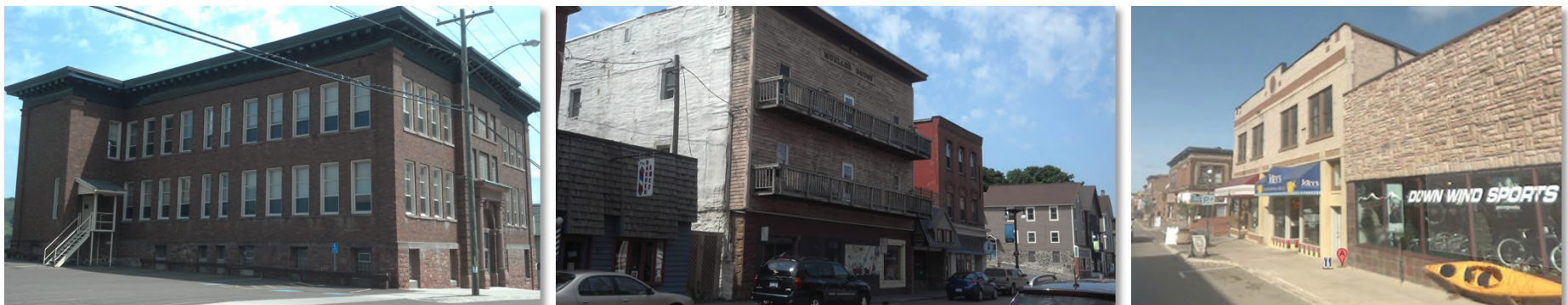
Left | St. Ignace School has recently been torn down.
