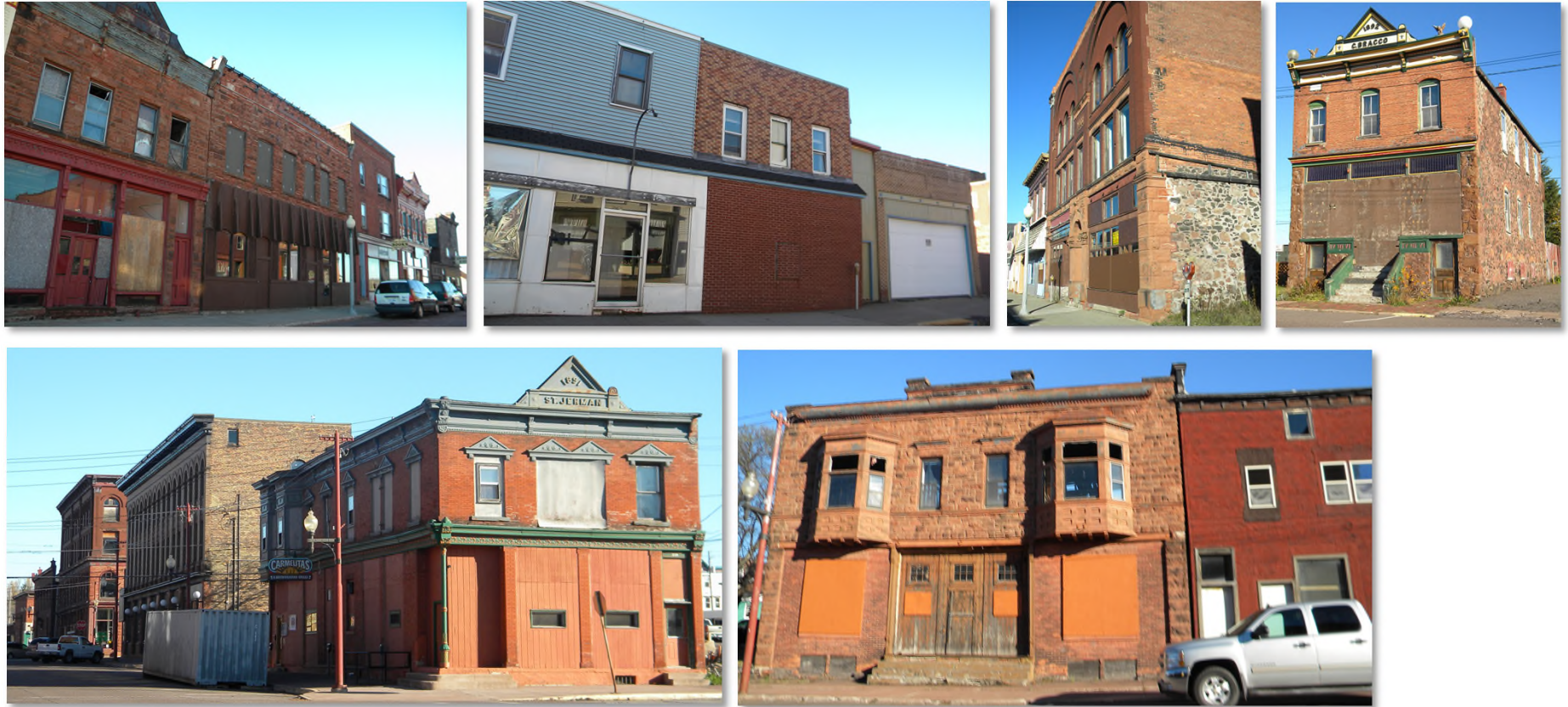
Photo credit (above): Original photos by LandUse|USA; 2016 © with all rights reserved.
