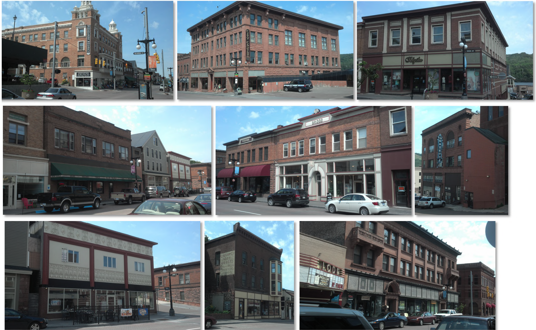
Photo credit (above): Original photos by LandUse|USA; 2016 © with all rights reserved.
