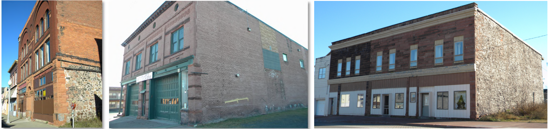
Photo credit (above): Original photos by LandUse | USA; 2016 © with all rights reserved.
